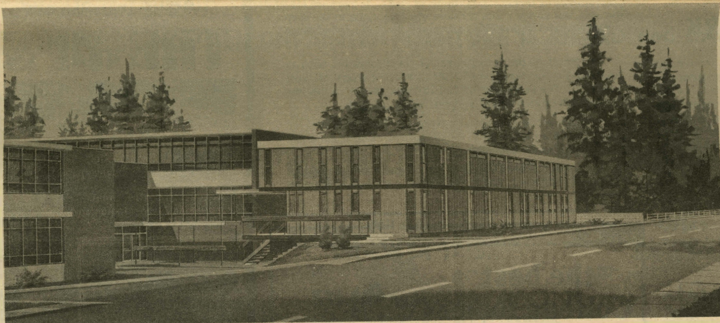
New administrative and library additions to Capilano College
