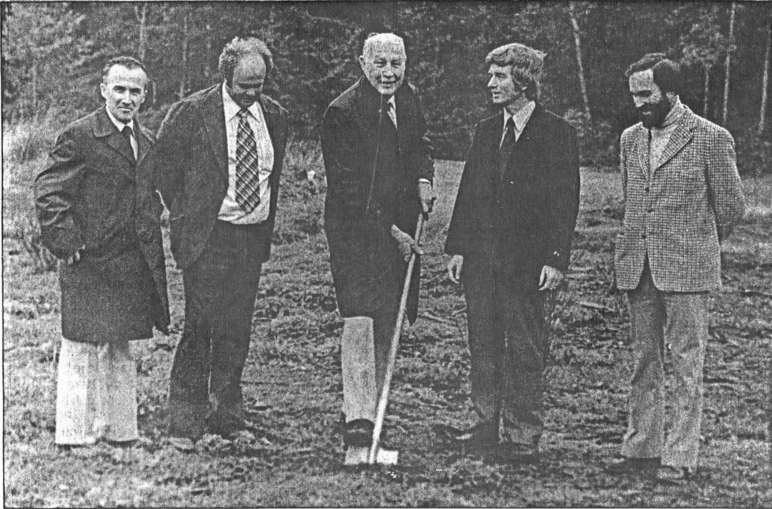
"There is still hope for society as long as we are turning the sod for buildings of higher learning." Those were the words spoken by Mayor Boucher of Sechelt as he turned over the ceremonial sod to mark the beginning of work on Capilano College. From left to right are Principal Paul Galliger, building owner Bill Van Westen, Mayor Boucher, College local representative Eric Paetkau, and Alex Smith, the Director of Planning. It is hoped that the College will be open by July.
