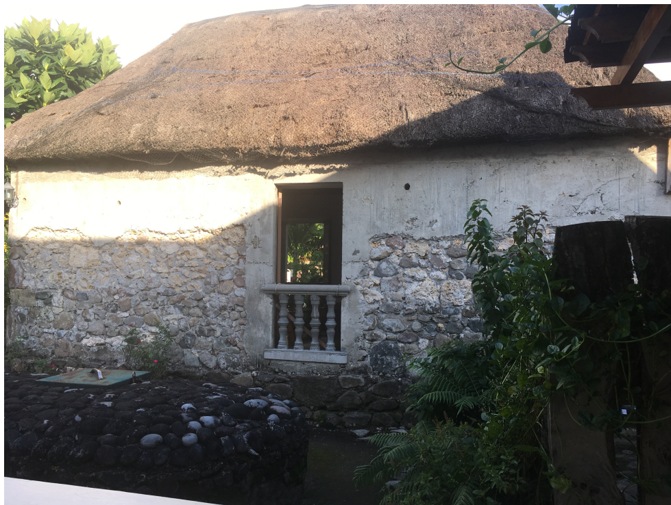
Figure 4. A sinadumpan in the above image in Itbud, Uyugan Municipality has a windowless wall on the headwind side to protect against strong gusts. The image below is a four-sloped roof maytuab in Basco, which is an improvement of the sinadumpan's two-sloped roof. Note the smooth wall masonry dividing the stone-exposed lower side wall, which ought to be the ideal finished design of traditional houses in the province. May 31, 2019.
